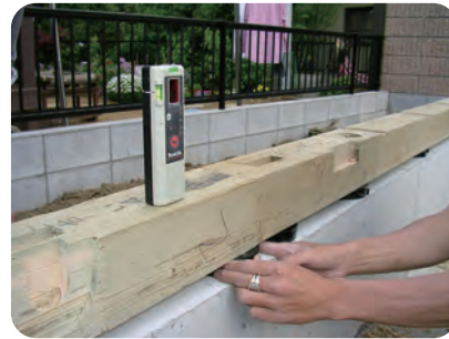
04 Turn adjustment claw of Relevel if there is a gap
