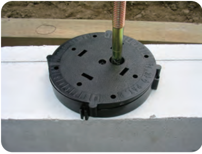
01 Put Relevel on slab level or floor
